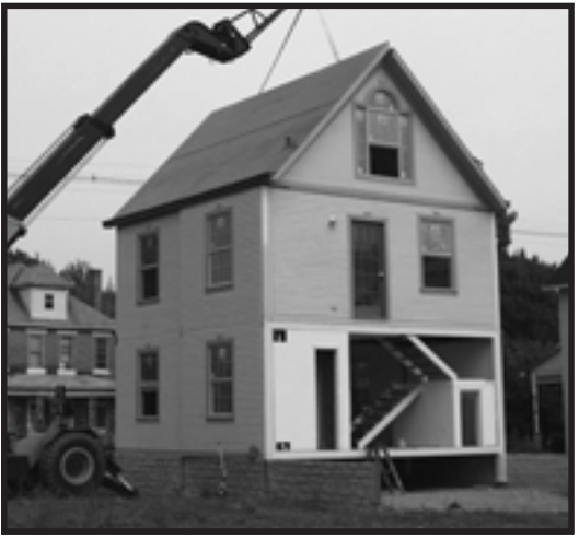
STEP 8: L2 & U2 (Lower & Upper roof sections)
