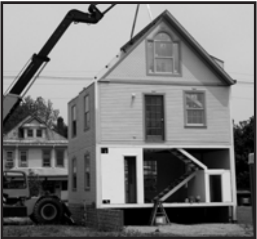
STEP 7: L1 & U1 (Lower & Upper roof sections)
