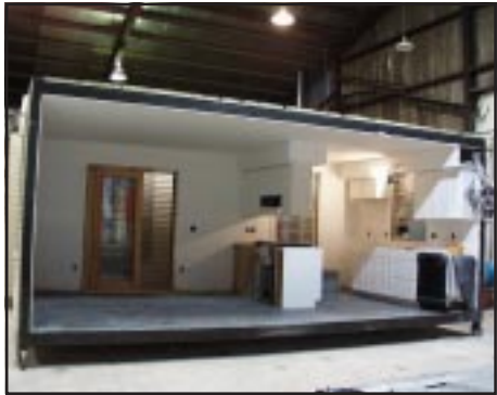
Kitchen (Cell C) prepared for flooring.
