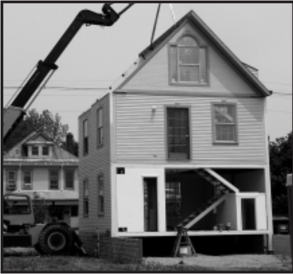
STEP 7: L1 & U1 (Lower & Upper roof sections)
