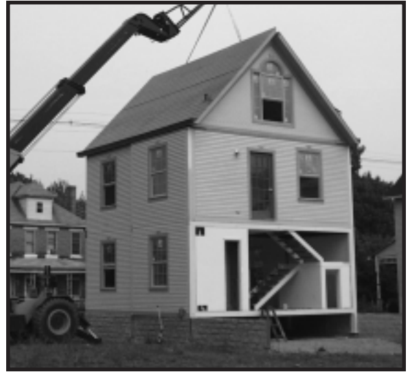
STEP 8: L2 & U2 (Lower & Upper roof sections)
