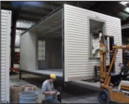
End wall adhesive and sealant installation.
