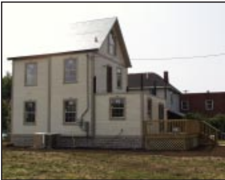
Side view, electrical hook-up. Weatherhead can be set-up for underground cable or traditional method, shown here, to blend with neighborhood.
