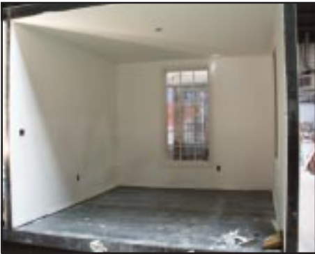
Carpet cut, cell ready for cleaning, switch and receptacle installation.
