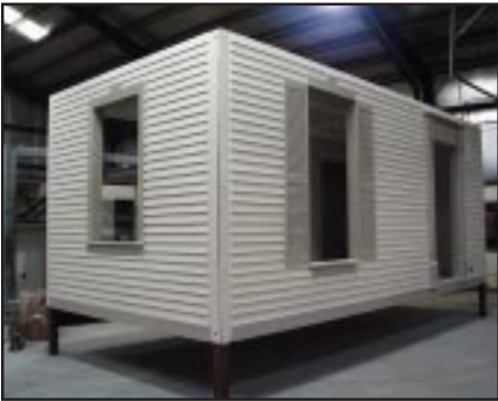
Installation of windows and door.
