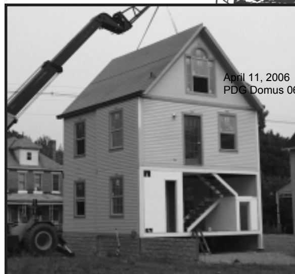
STEP 8: L2 & U2 (Lower & Upper roof sections)
