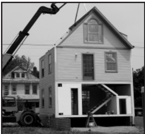
STEP 7: L1 & U1 (Lower & Upper roof sections)
